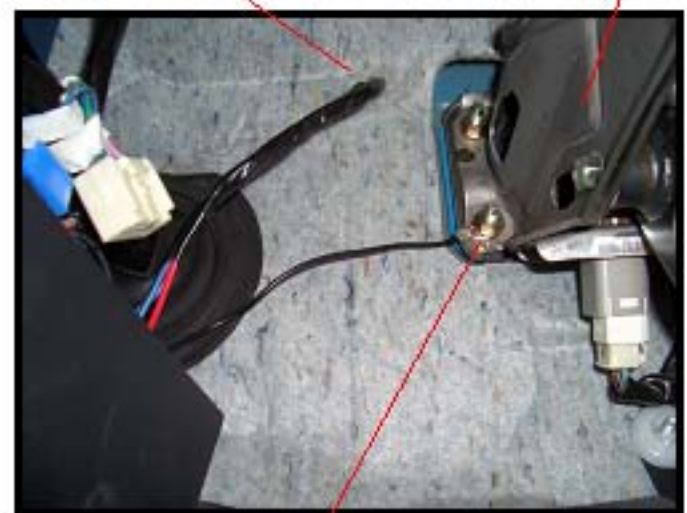
Switch ground connection
